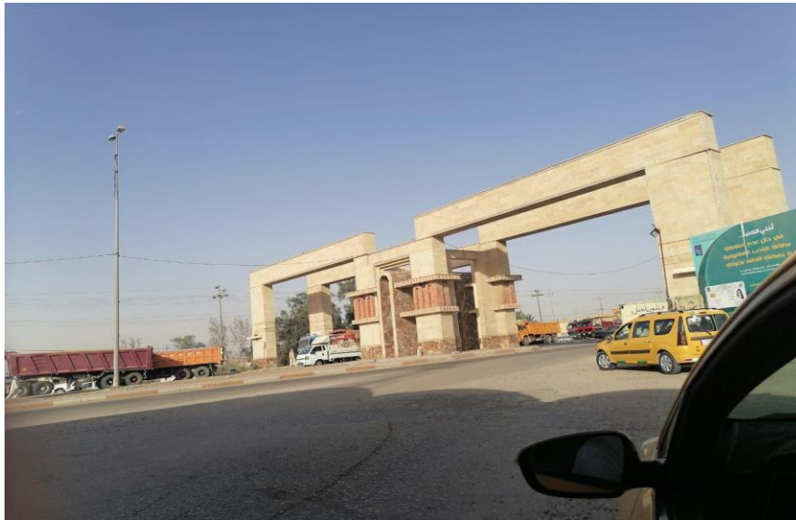
Picture (1), south entrance, silo control
