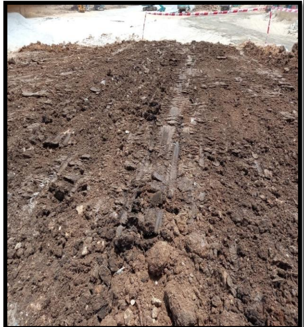
Spreading of Clay Soil at Top Surface
