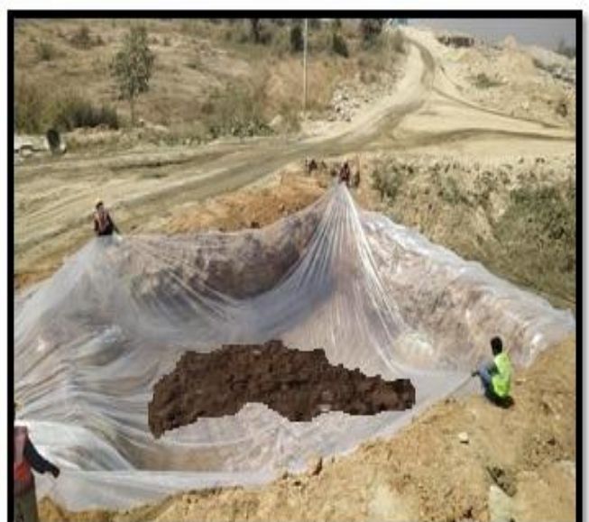
Spreading of Impervious layer at km :97+000 for disposal of bituminous waste
