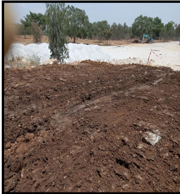
Spreading of Clay Soil at Top Surface
