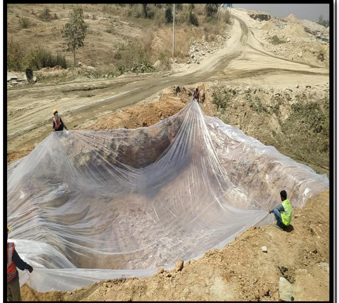
Spreading of Impervious layer at km :97+000 for disposal of bituminous waste
