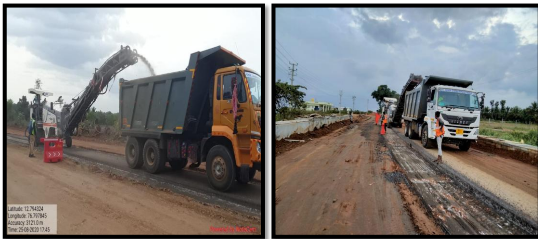
Figure Shows the Photograph for Extracting of Milling Material from Existing Road.
