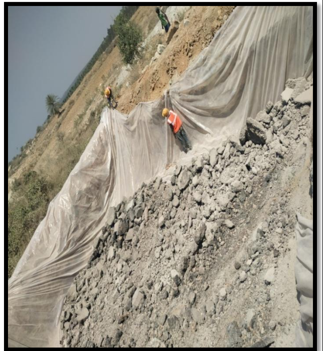
Photo Showing Debris Dispose to Prepared Pit
