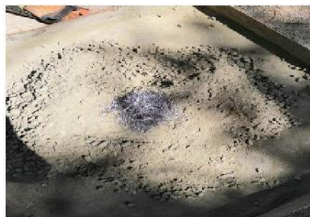
Casting and curing of test specimens
